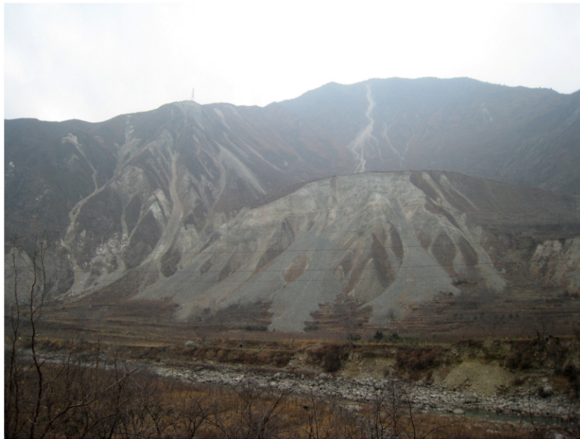
Fig. 19. Shallow landslides occurred in eluvium and colluvial layer of slopes (with camera direction of 290°).
